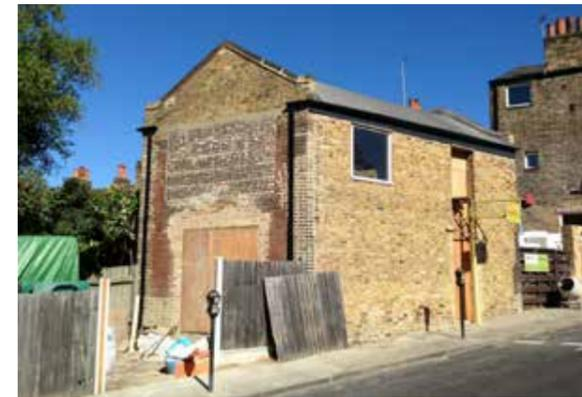
Ecomerchant customer Roger Nelson wanted to convert an outbuilding at his house in the center of Greenwich built around 1830 into a living space and studio. The buildings are of soft London brick, and lime mortar with solid 9 inch walls. Although not listed it is in a conservation area, which meant all changes required planning approval and the external appearance would have to be largely unchanged.
