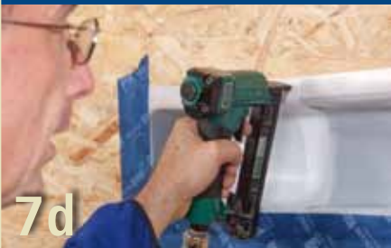
Enlarging: Fixing the overlap
