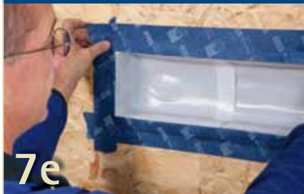
Enlarging: Bonding
