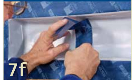
Enlarging: Taping over the overlaps
