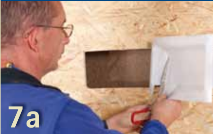
Enlarging: Cutting to size
