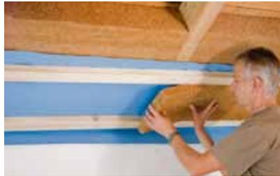
With this solution the weather tightness of the structure is not affected and there is no need for scaffolding.
