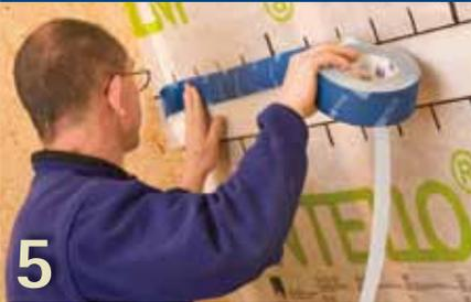
**5** Place TESCO VANA centrally over the overlap, unroll and stick down over the joint piece by piece. Press firmly to secure the tape, ensuring there is sufficient back-pressure.
