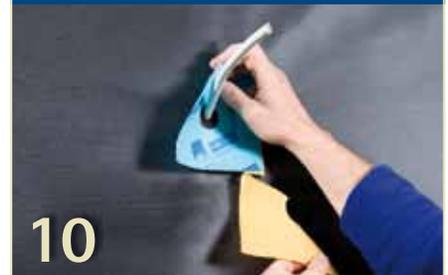
**10** Sealing around holes with KAFLEX or ROFLEX EPDM grumets or collars. Tape over KAFLEX (self-adhesive) using TESCO VANA or INVIS to seal outdoor joints. Stick down ROFLEX using TESCO VANA or INVIS. Press firmly to secure the adhesive tape.
