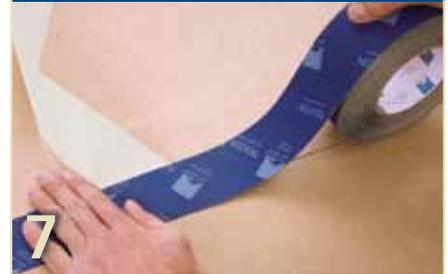
**7** Use TESCO VANA for sub-roofs made of wood-based panels (ie. GUTEX). Place the tape centrally over the butt joint, unroll and stick down over the joint piece by piece. Press firmly to secure the tape. Prime softwood fibre panels with TESCO PRIMER RP.
