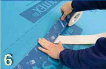
**6** Use TESCO VANA to join roof lining membrane (e.g. pro clima SOLITEX). Place the tape centrally over the overlap, unroll and stick down over the joint piece by piece. Press firmly to secure the tape, ensuring there is sufficient back-pressure.
