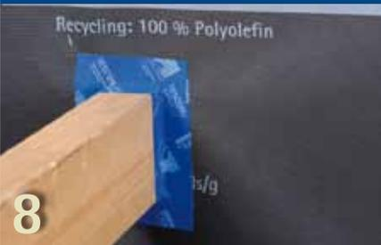
**8** Making a windtight and water tight joint to planed rafters or roof beams with TESCO PROFIL. Bonding sequence: 1st bottom, 2nd left and right hand sides, 3rd top. Make airtight joints indoors in the same way.
