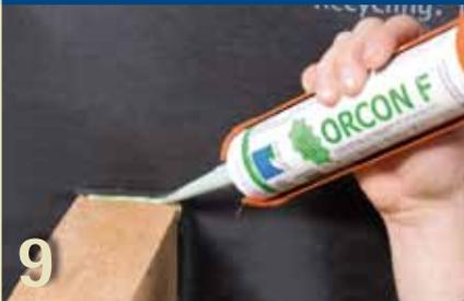
**9** Use ORCON F joint adhesive on unplaned rafters or roof beams, applying a continuous bead approx. 5 mm thick (more may be needed on rough substrates).
