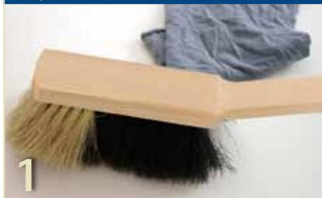
All surfaces must be stable, dry, smooth and free of dust, silicone and grease. Sweep or vacuum clean and wipe all surfaces.
