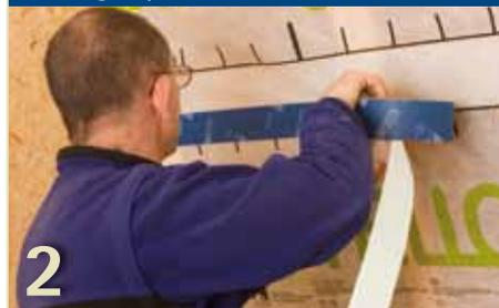
Place the TESCO VANA centrally over the overlap, unroll and stick down over the joint continuously. Press firmly to secure the tape, ensuring there is sufficient back-pressure.
