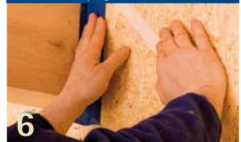
Seal corners using pro clima TESCO PROFIL corner sealing tape. Remove one strip of the split release paper and press down the first piece. Then remove the second strip of the release paper and press down the second piece.
