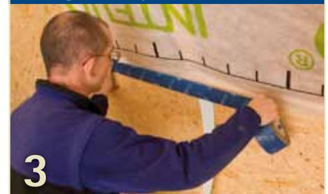
To create airtight joints between vapour checks and smooth, non-mineral surfaces such as wood-based panels or planed wood, place TESCO VANA centrally over the joint, unroll and stick down over the joint continuously.
