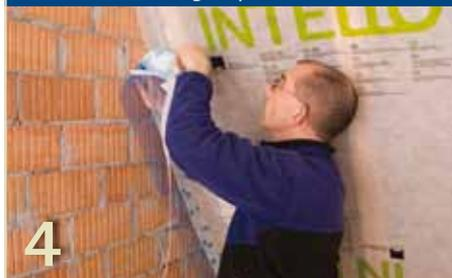
Use pro clima CONTEGA PV for reliable joints to gypsum based plaster. Affix fleece to the membrane with tape and use ORCON F to affix it to the masonry at intervals. Embed the reinforcement and the fleece in the middle layer of gypsum based plaster.
