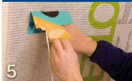
Seal all round penetrations with EPDM grommets. Cable grommets have a self-adhesive. Stick pipe grommets to the substrate with TESCO VANA to form an air-tight seal. Press firmly to secure the adhesive tape.
