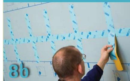
Alternatively, it may be sufficient to place strips of tape no more than 30 cm apart to relieve the load. However a supporting lath is the optimum recommendation.
