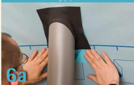
Pull a pro clima EPDM pipe grummet over the pipe and create an airtight seal between it and the airtight sealing layer using UNI TAPE.
