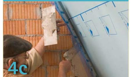
Apply and smooth gypsum based plaster behind the fleece and reinforcement layer. Insert the fleece and reinforcement layer and then cover completely with gypsum based plaster.
