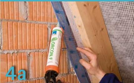
Use pro clima CONTEGA PV for reliable joints to gypsum based plaster. Affix the fleece to the masonry at intervals using ORCON F. Please note: Ensure the tape is flat and does not have any voids or bubbles!
