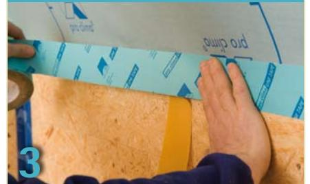
To create airtight joints between vapour checks and smooth, non-mineral surfaces such as wood-based panels or planed wood, place UNI TAPE centrally over the joint, unroll and stick down over the joint continuously.
