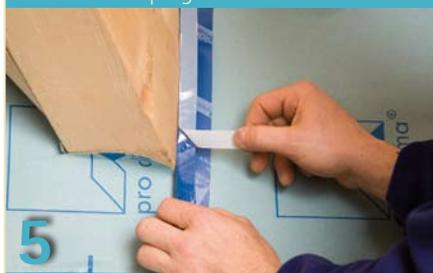
Join corners using pro clima TESCO PROFIL corner tape. Remove one strip of the split release paper and press down the first piece. Then remove the second strip of the release paper and press down the second piece.
