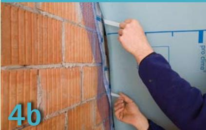
Apply the vapour check. Remove the release paper from the back of the CONTEGA PV and affix the fleece to the airtight sealing layer using integral adhesive tape. Press firmly to secure.
