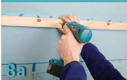
If using blow-in insulation materials, secure the tape over overlaps with a supporting lath. Only use appropriate vapour checks (e.g. DB+ or intello plus).
