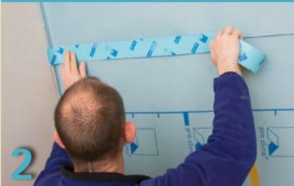
Place the UNI TAPE centrally over the overlap, unroll and stick down over the joint continuously. Ensure there is sufficient back-pressure. UNI TAPE 40 mm is only suitable for use on hard surfaces (e.g. OSB).
