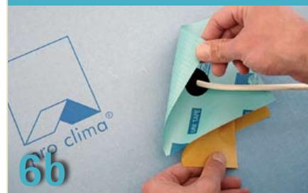
Seal cables using self-adhesive cable grummetts. Pull the cable through, remove the release paper, affix the grummet and press firmly to secure.
