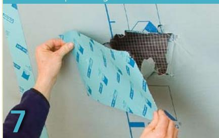
Use pro clima UNI TAPE XL (15 or 20 cm wide) for patching repairs. Press firmly to secure the tape, ensuring there is sufficient back-pressure.
