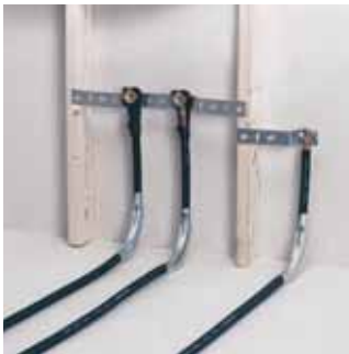
First fix bath tap and W.C. fittings
