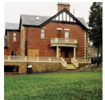
Prestigious Refurbishment Project
