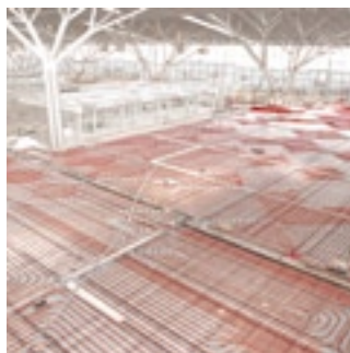
REHAU Underfloor Heating system
