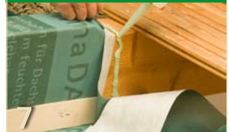
Joints to sub-and-top membrane
