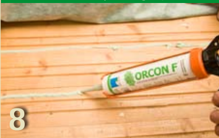
Joints to outer airproofing layer
