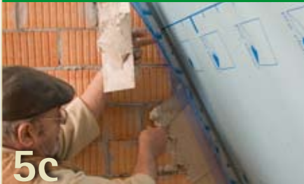
Joints to unplastered walls
