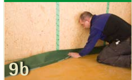
Joints to wall or concrete floor slab
