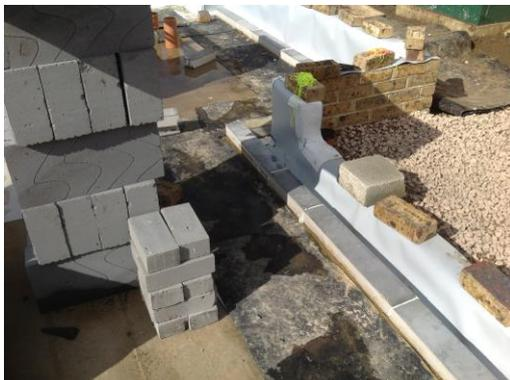
To meet the demands of the Code, insulation increases on the walls, floors, windows etc which can leave the thermal bridge at the wall floor junction a weak link in the chain. Proportionately, heat loss through this thermal bridge can account for about 5 to 7% of the total heat loss of a well-insulated building.
