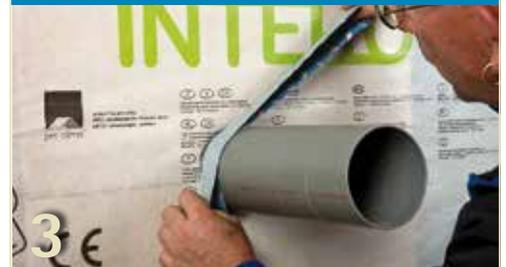
Place the tape on the tube and tape it around the tube gradually. Ensure sufficient coating of the ends.
