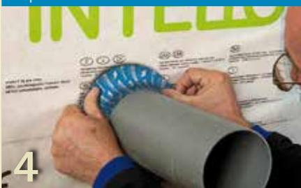
Remove the second release paper completely. Gradually fold the tape onto the surface and piece by piece tape it all around.
