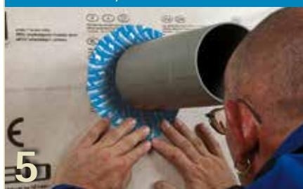
Afterwards, press bonding firmly all around. Ensure there is sufficient back-pressure. The pressing aid pro clima PRESSFIX is particularly efficient and protects your hands.
