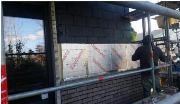
Blowerproof can be applied on the inside or the outside as long as it is applied on the warm side of the insulation. See picture left.
